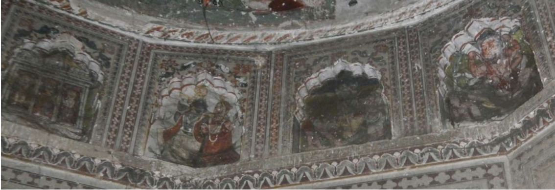
Figure 14: Niches with Avatara Panels
