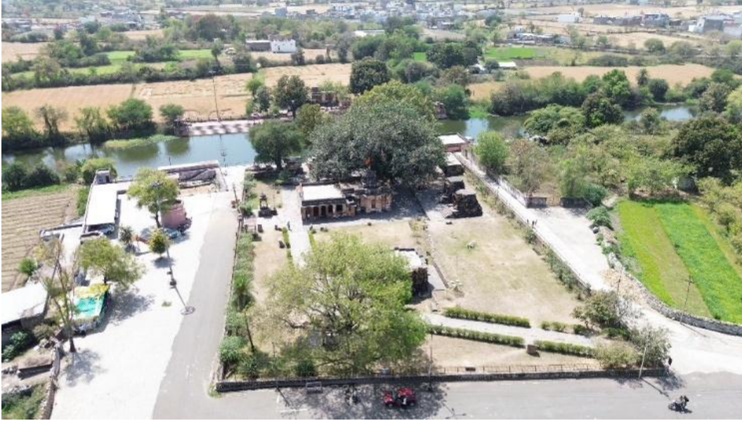
Figure 31 An aerial view
