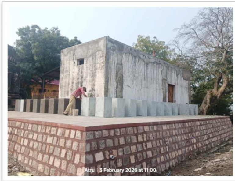
Work of construction of a new larger sculpture shed and upgradation of existing sculpture shed at Ganesh Mandir, Atru in progress
