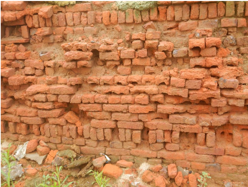
Pl. 5. Kushan period brick used in a modern wall, Jahangarh.
