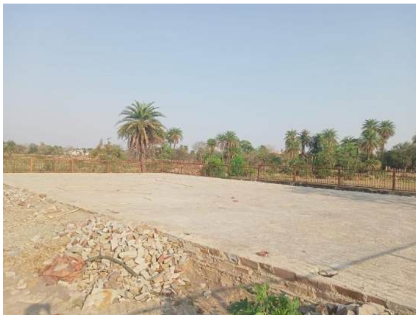
Foundation base prepared at Bijolia
