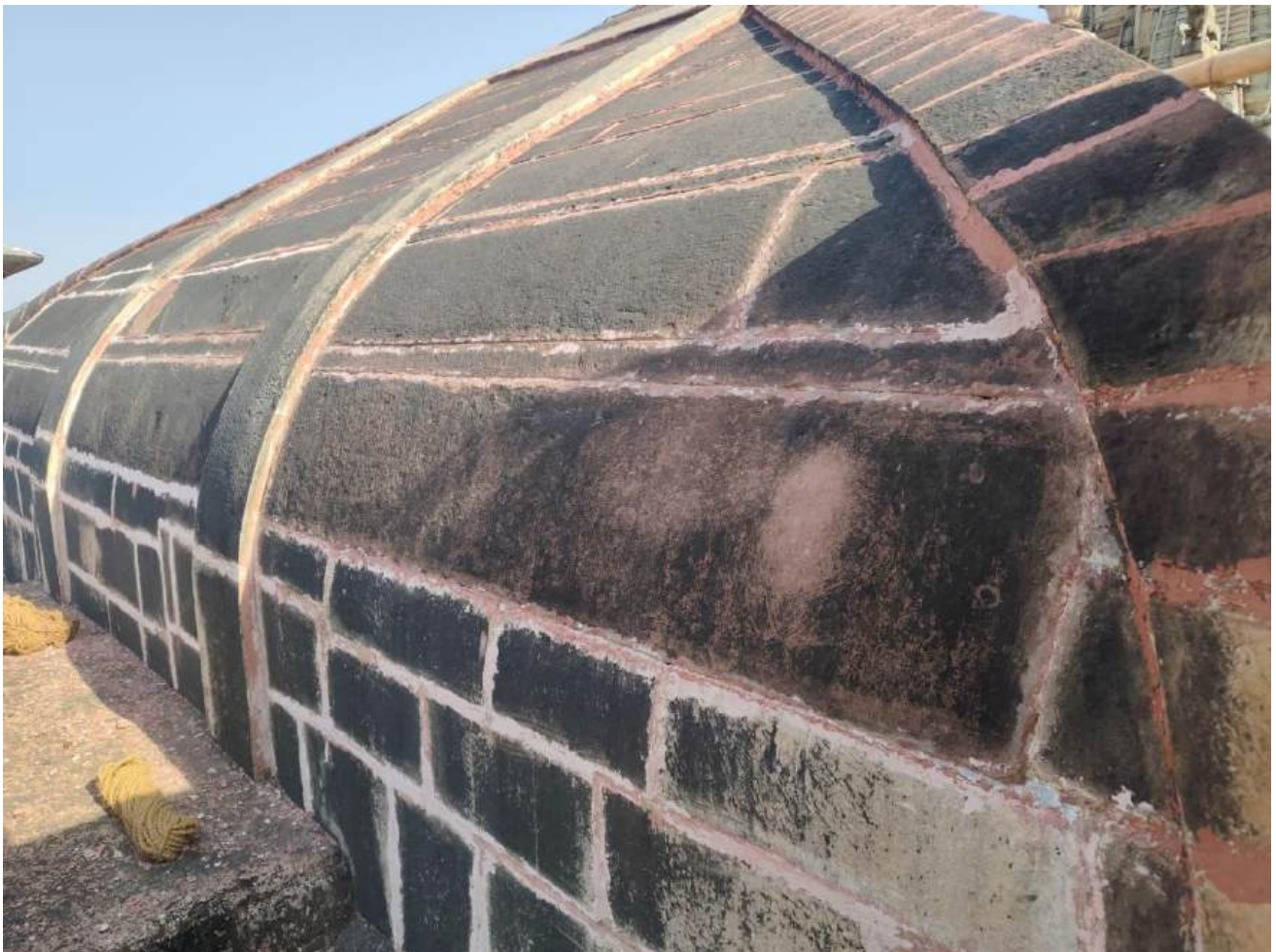
Recess pointing work at top of ceiling
