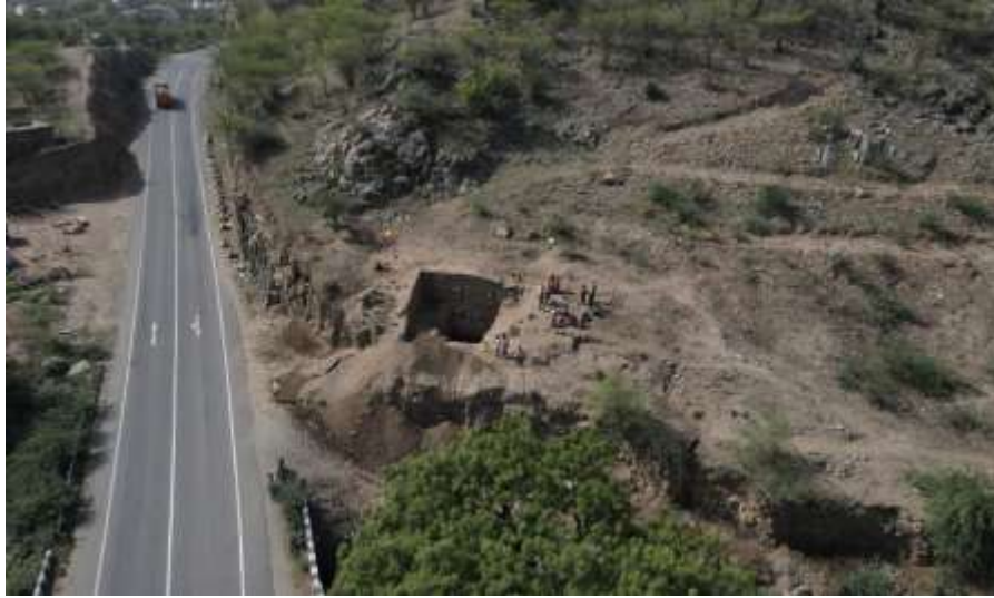
Pl. 7. An aerial view of trench
