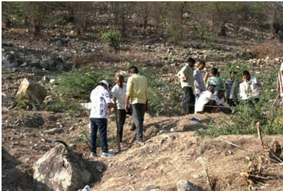
Pl. 8. Laying-out of trench
